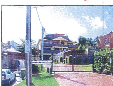
Residential Building in Maroomba Rd
