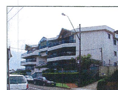
residential units on corner
